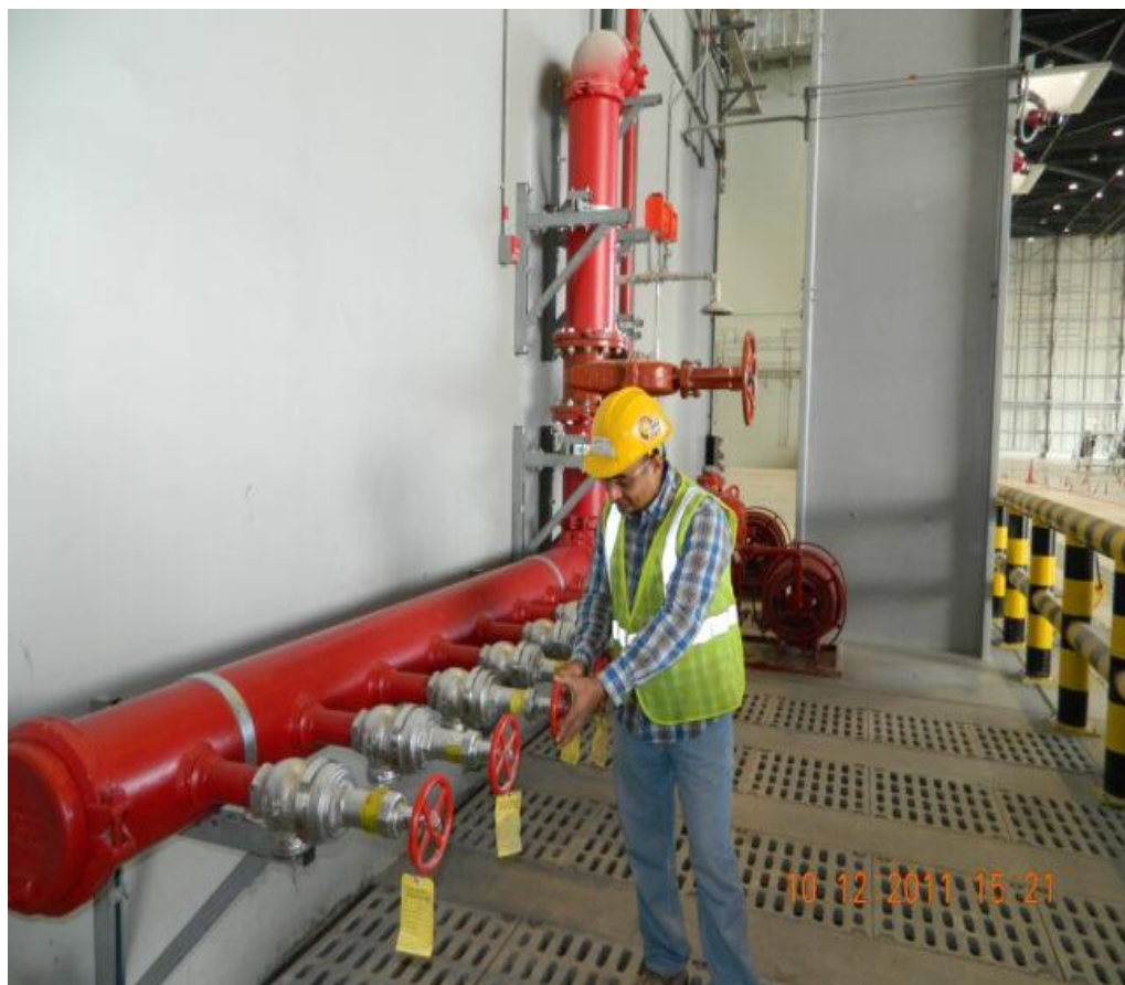
Nasirhusen Lotiya. Fire Safety Inspection.
