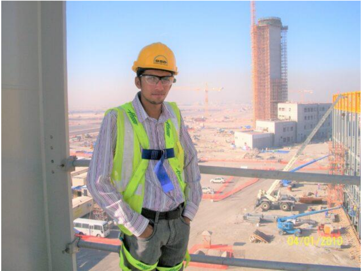
Matin Manman conducting roof inspection of the Cargo Terminal Hamad International Airport – Doha, Qatar
