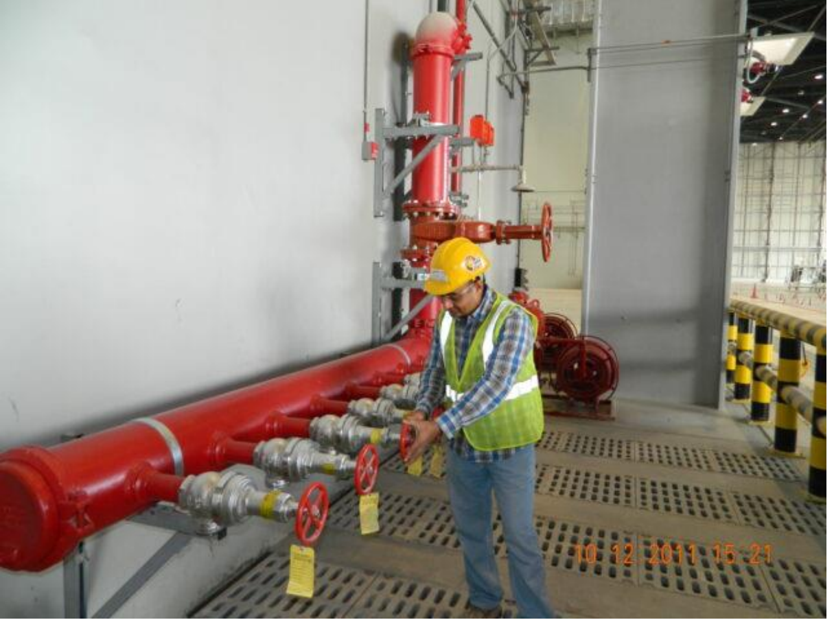
Nasirhusen Lotiya. Fire Safety Inspection.
